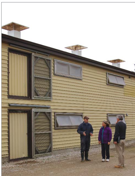
Glen MacArthur (l.) demonstrates how retrofitting an existing barn with a natural ventilation system – including the roof exhaust vents and sidewall air inlets shown – cuts energy costs.
